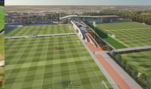
COLUMBIA PARK TRAINING FACILITY
